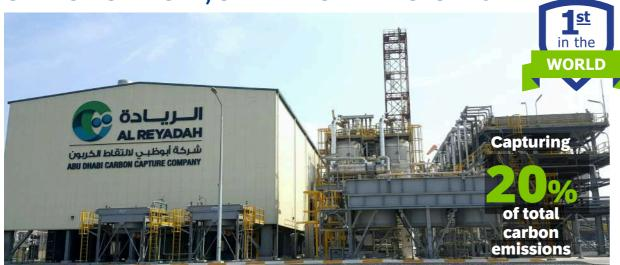
Emirates Steel in partnership with ADNOC & Masdar has developed world's first **CCUS for steel production.** With capacity of up to 800kt of CO2/year and pipe it 43 km to ADNOC's Rumaitha and Bab oil fields. System is working since 2016.
