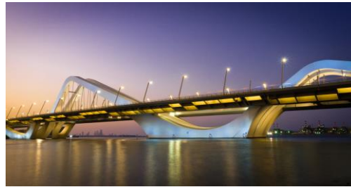
Sheikh Zayed Bridge
